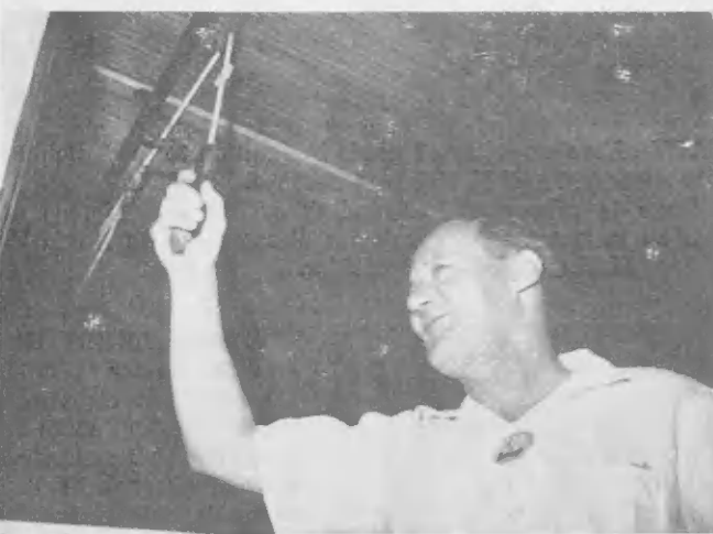
A WOODEN tool called a fid is used to open up rope while splicing. Performing this ancient, yet still effective, task is Julio Dorothal, center, Mechanical-Yard stevedore corporal, who has thirty-one years' service.
